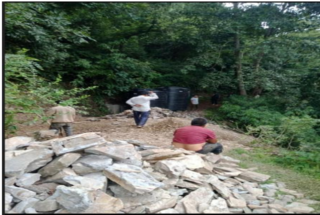
Figure: Excavation, Soling work for downstream reservoir tank
